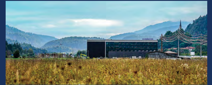
Hamilton Storage Headquarters Located in Domat/Ems, Switzerland.
