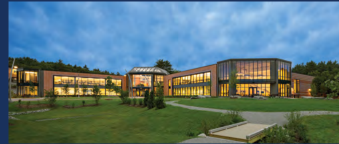
Hamilton Storage Headquarters Located in Franklin, Massachusetts, USA.
